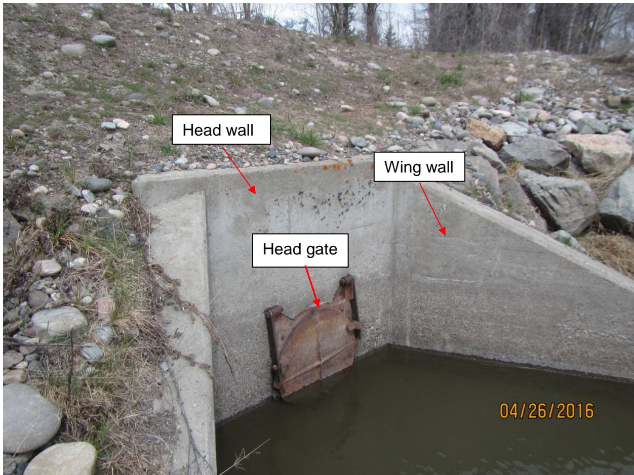
Figure 2-4. Flapper-type head gate on drainage culvert.
