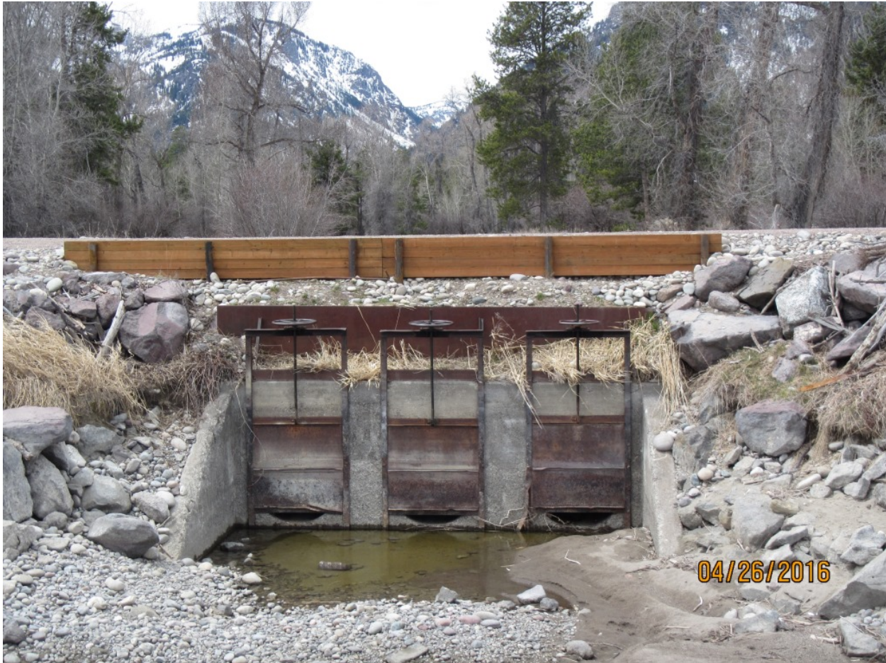
Figure 2-5. Manually operated head gates on an irrigation intake culvert.
